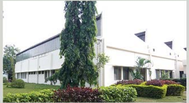
Hydraulic Pumps & Motors Plant
