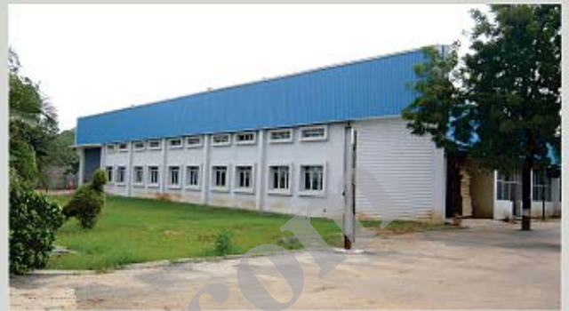
Hydraulic Valves Plant
